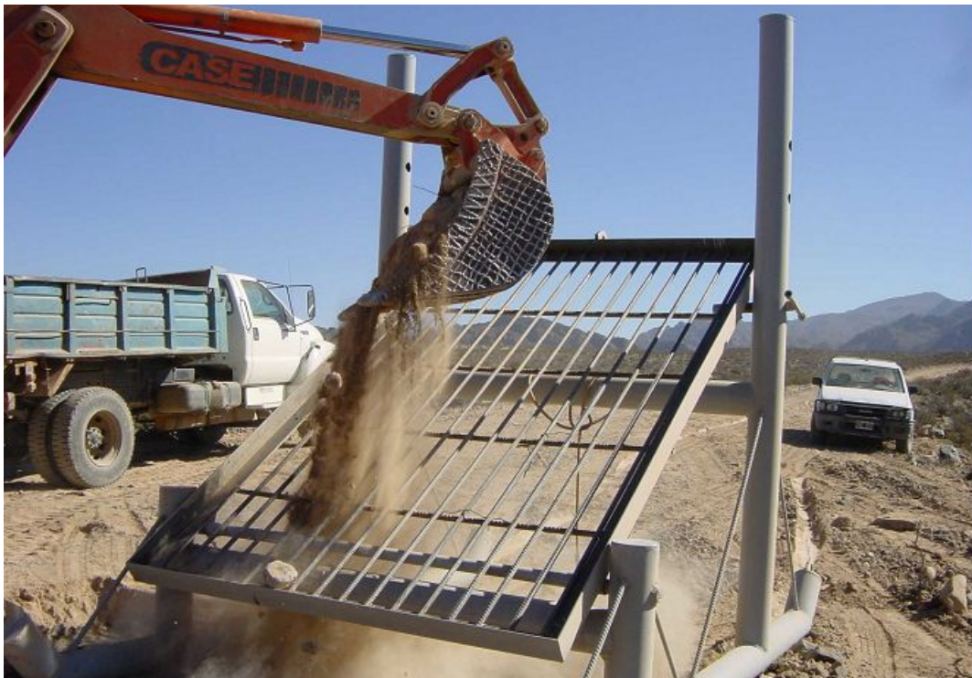
Figure 2.2 Large-scale field screen (grizzly) used to remove material greater than 100 mm.
