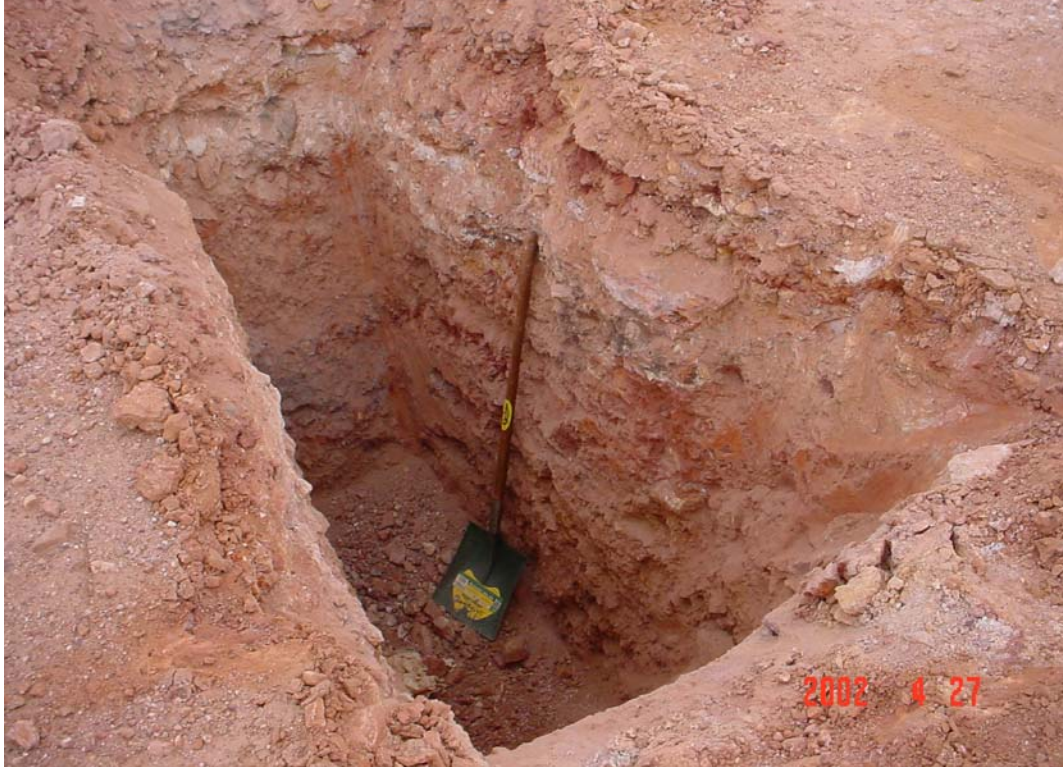
Figure 2.1 A 2.0 m test pit excavated in waste rock material.
